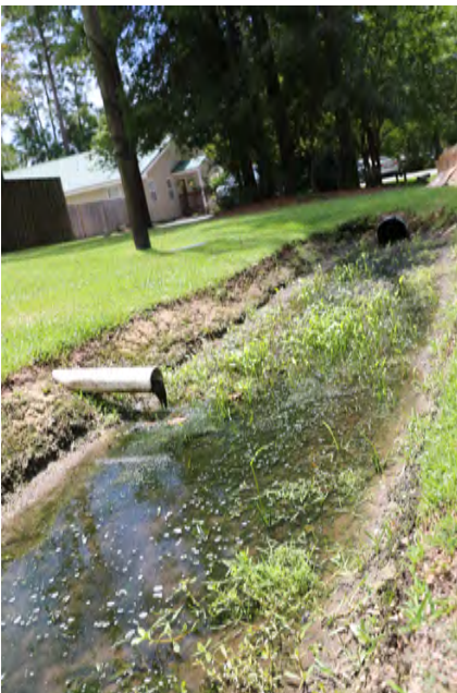
Sewage polluted roadside drainage ditch with drain pipe from an OSDS.
